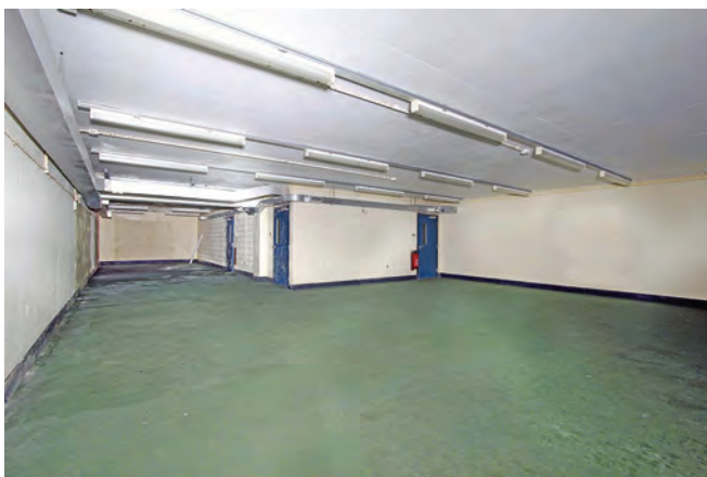
The L-shaped government departments room on the upper floor. This is one of the largest rooms in the bunker
